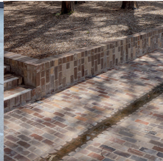
RW: Brick retaining wall
